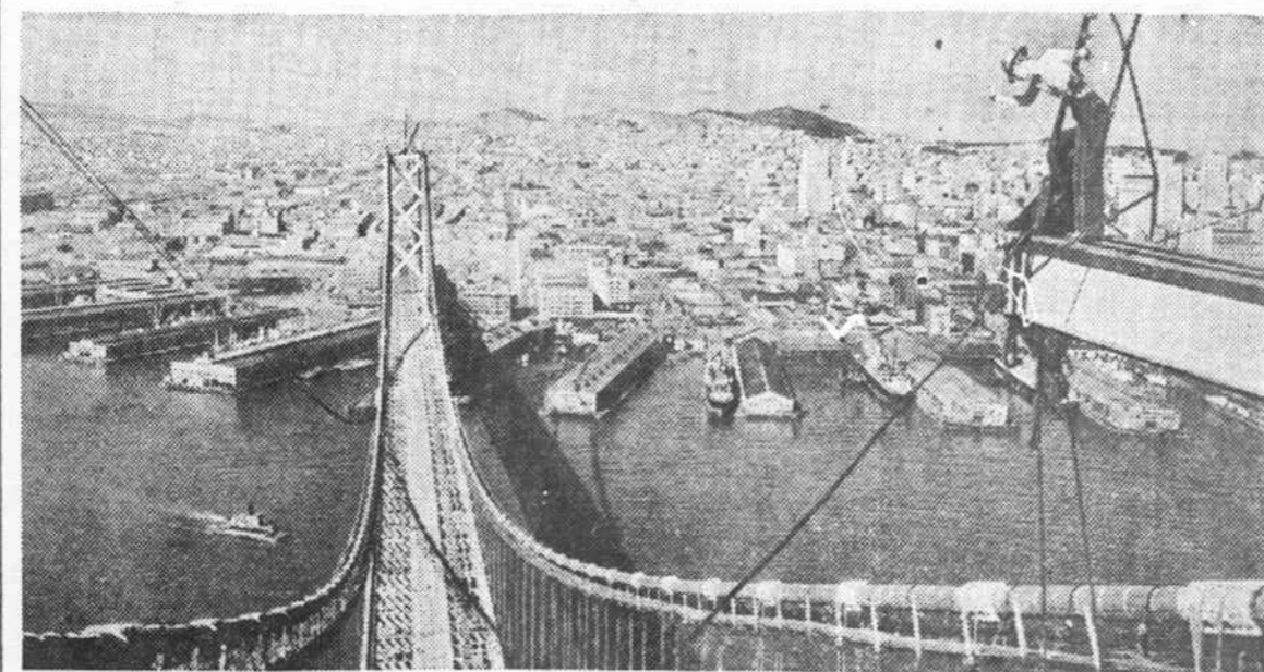
Automobiles will be passing over the San Francisco-Oakland Bay bridge by next November, engineers predict. The view shows the center lane with the floor steel entirely erected on the West Bay Crossing. The bridge, largest structure of its kind in the world, will cost $77,200,000 on completion.
