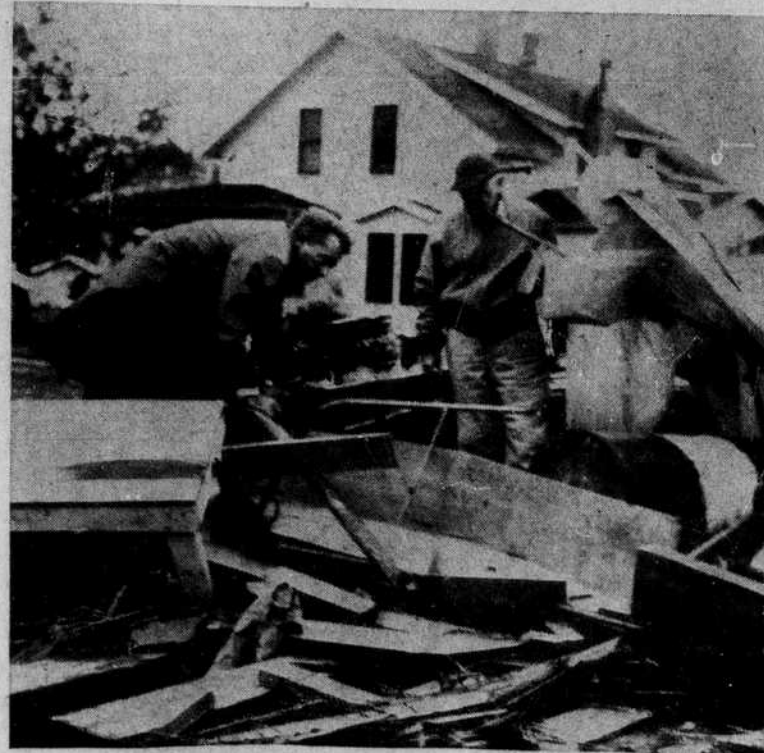
SURVEY—Waters Thompson, left, and his father, R. L. Thompson, survey the wreckage of their Esso Marine Dock, which is piled up on Moore Street beside the H. T. St George home following the storm.—(Photo by Art Newton.)
