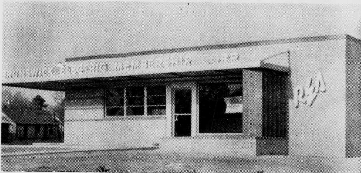
MODERN IN DESIGN, and designed for functional efficiency, is the Brunswick Electric Cooperative's branch office in Whiteville. The Co-op only last week occupied the $65,000 plant, and is open now for business there. It is located at 307 South Lee Street.
