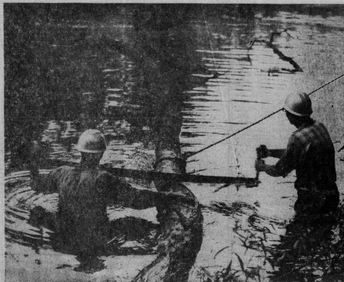
LAST LAP —Orb Duncan, left, and Brazton Generette, standing waist deep in water, get busy on the last lap of the Brunswick-Columbus stream clearance project that has been in progress for the past several months. Great improvement in drainage in several areas has resulted.—(Corps of Engineers photo.)
