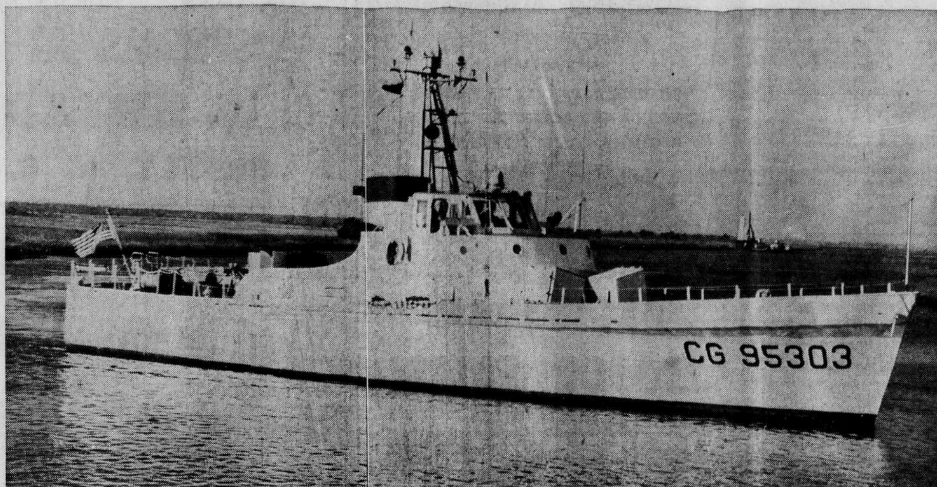
ARRIVES —This is the new Coast Guard patrol boat, which arrived at her new station in Southport last week. She is a 95-foot vessel and takes the place of the old 83-footer which has been based here for the past several years. The new patrol boat
