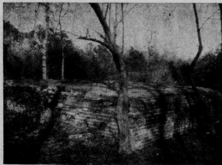
TOMB —One of the most unusual burial arrangements in the history of Brunswick County is the Gause Tomb, which is located in the woods about a mile from the site of the old Gause Manor at Gause Landing. The burial vault is of masonry construction, with brick walls 18-inches thick. The structure is about three feet high, but extends about that same depth below the ground. It is 15x15-feet, and is well preserved, except for a hole blasted at one corner by vandals.
