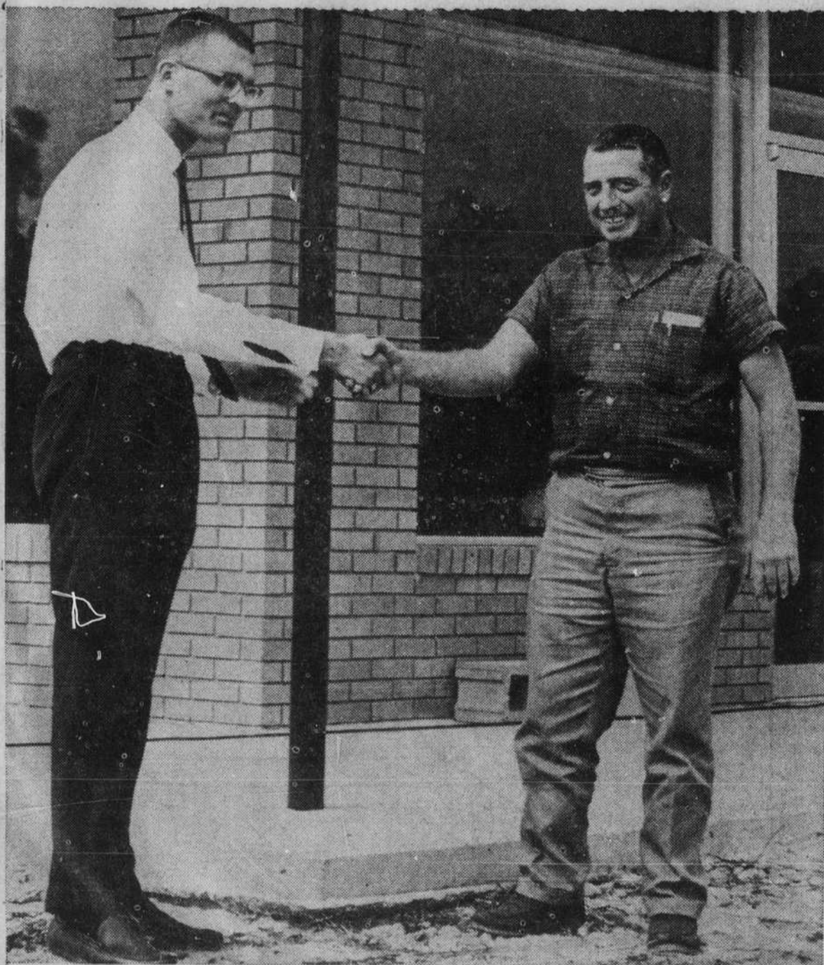
COMPLETED—Hal Reeves, left, congratulates Jim Hufham, right, upon the completion of his new Shopping Center building at Boiling Spring Lakes. It will be open for business for the first time during the big promotion that is scheduled for the weekend of October 19-21 at the big residential development near Southport.
