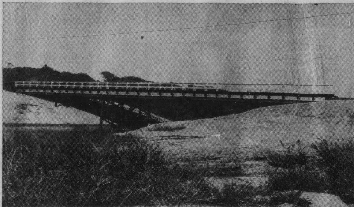
COMPLETED —This is the new bridge crossing Davis Creek between the Tranquil Harbour section and the strand at Long Beach. The street has been paved and now affords hard surface travel through both sections. (Staff Photo by Allen)
