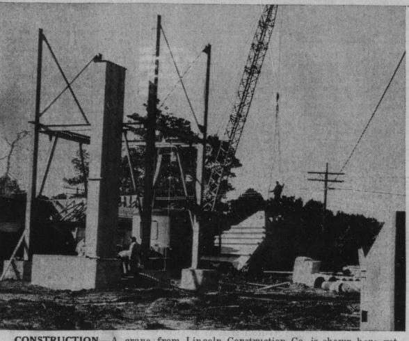
CONSTRUCTION-A crane from Lincoln Construction Co. is shown here getting ready this morning to lift the giant hopper in place for the new ready-mix concrete plant, a new facility for Blake Construction Co in Southport. The plant is expected to be in operation within a few day. (Staff Photo by Allen)
