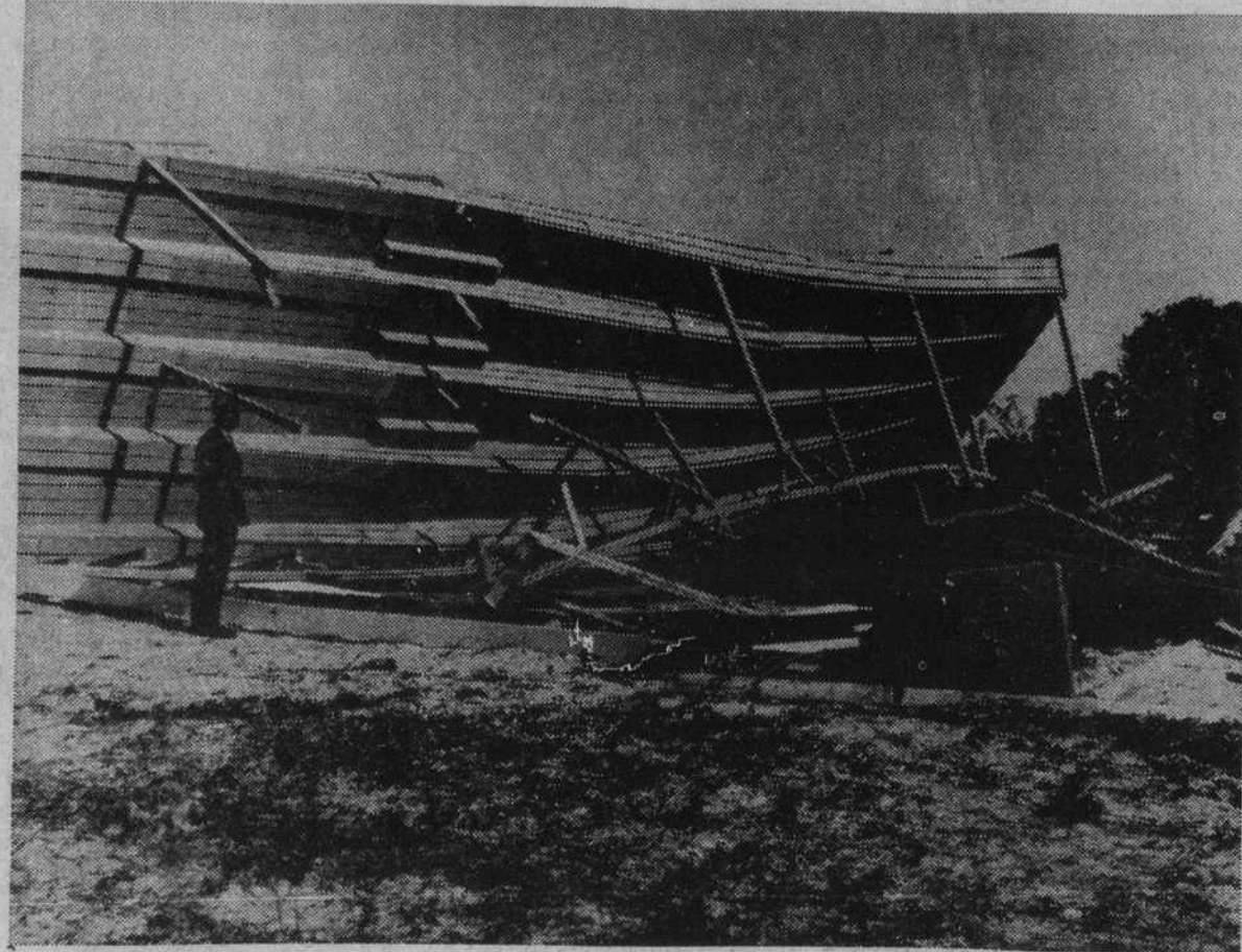
WRECKED —BCT Coach Anthony Davis is shown standing in front of the grandstand at the school's athletic field after it had been toppled over and demolished by the force of a heavy windstorm Sunday morning. (Staff Photo by Allen)
