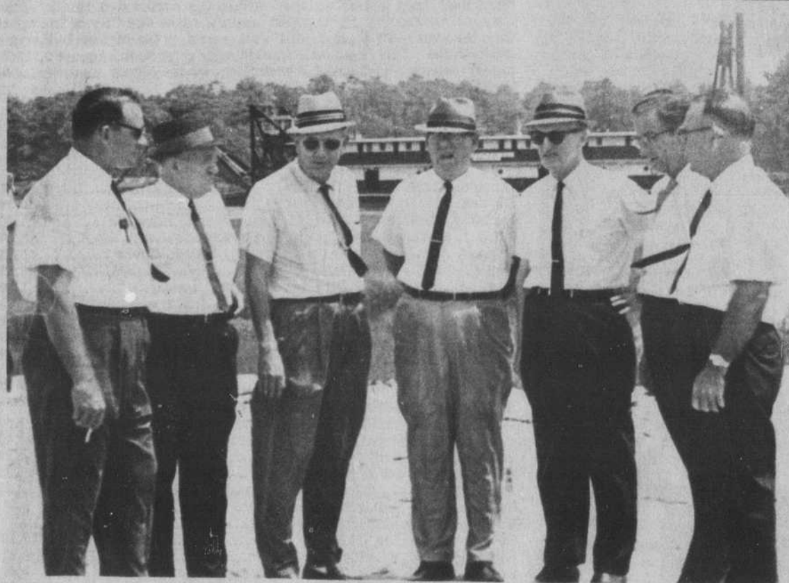
Visit To Ferry Site
