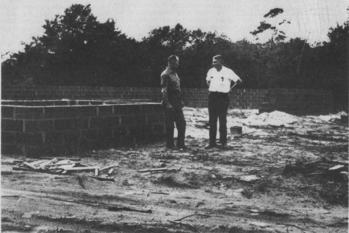
New Building Going Up
