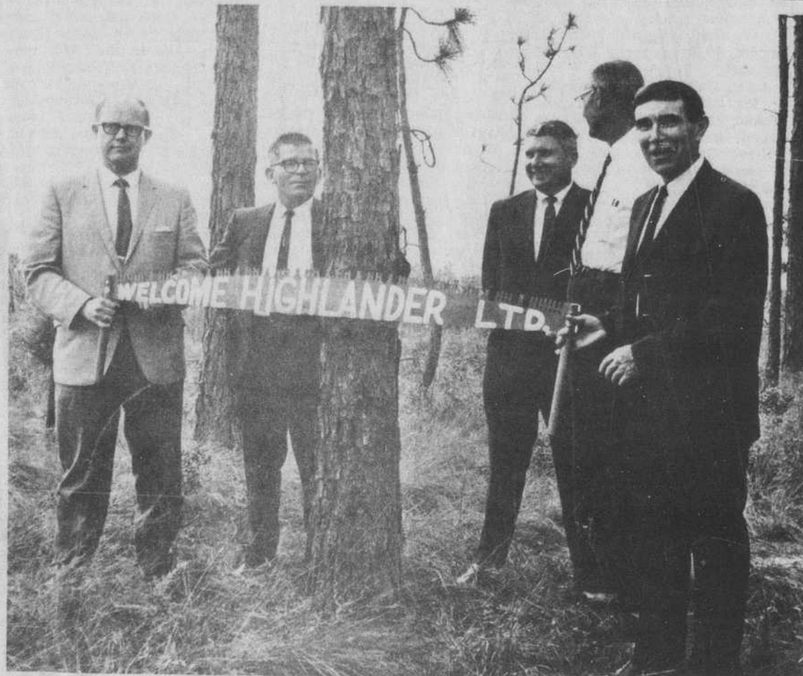
Tree Cutting For New Industrial Building
