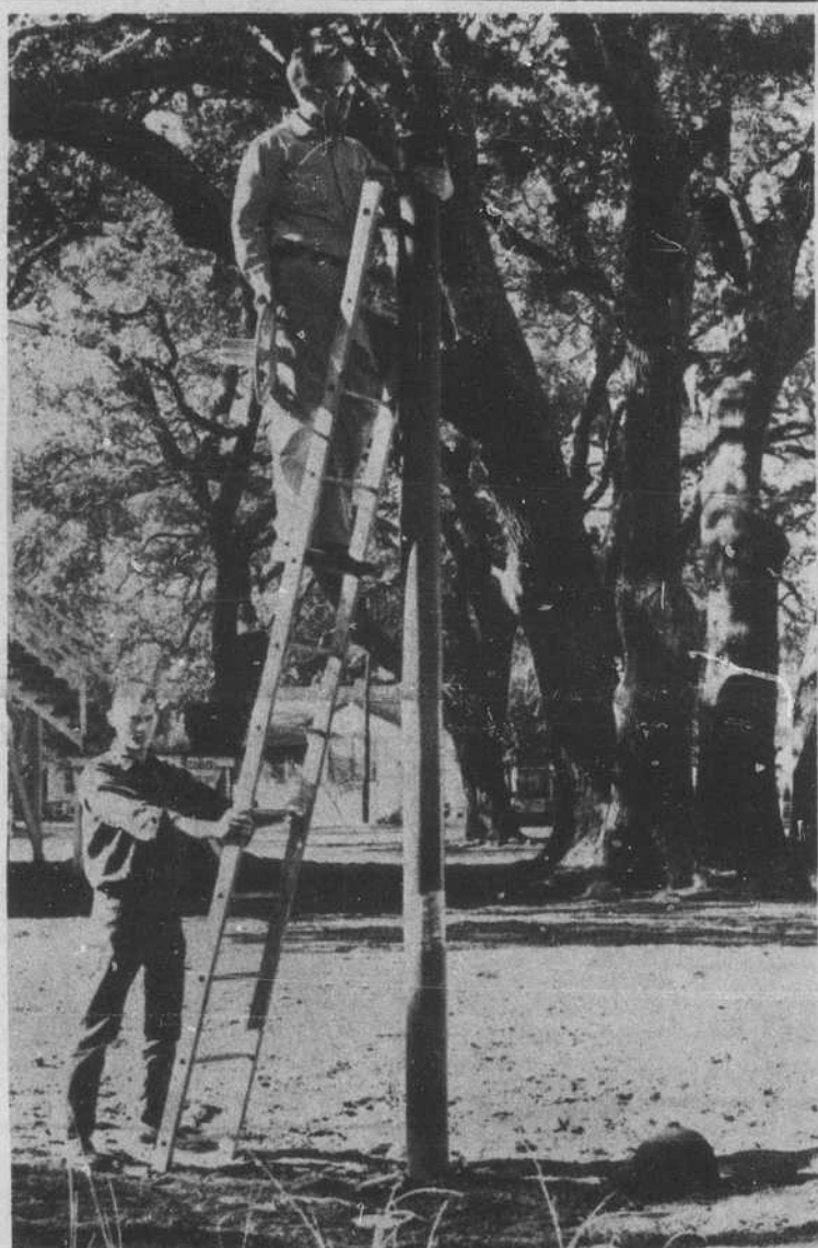
Repair Playground Equipment
