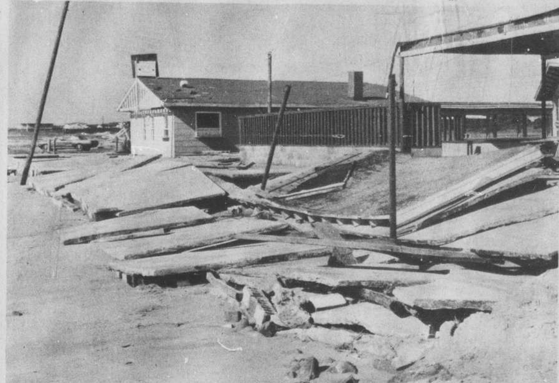
Waterfront Damage At Yaupon Beach
