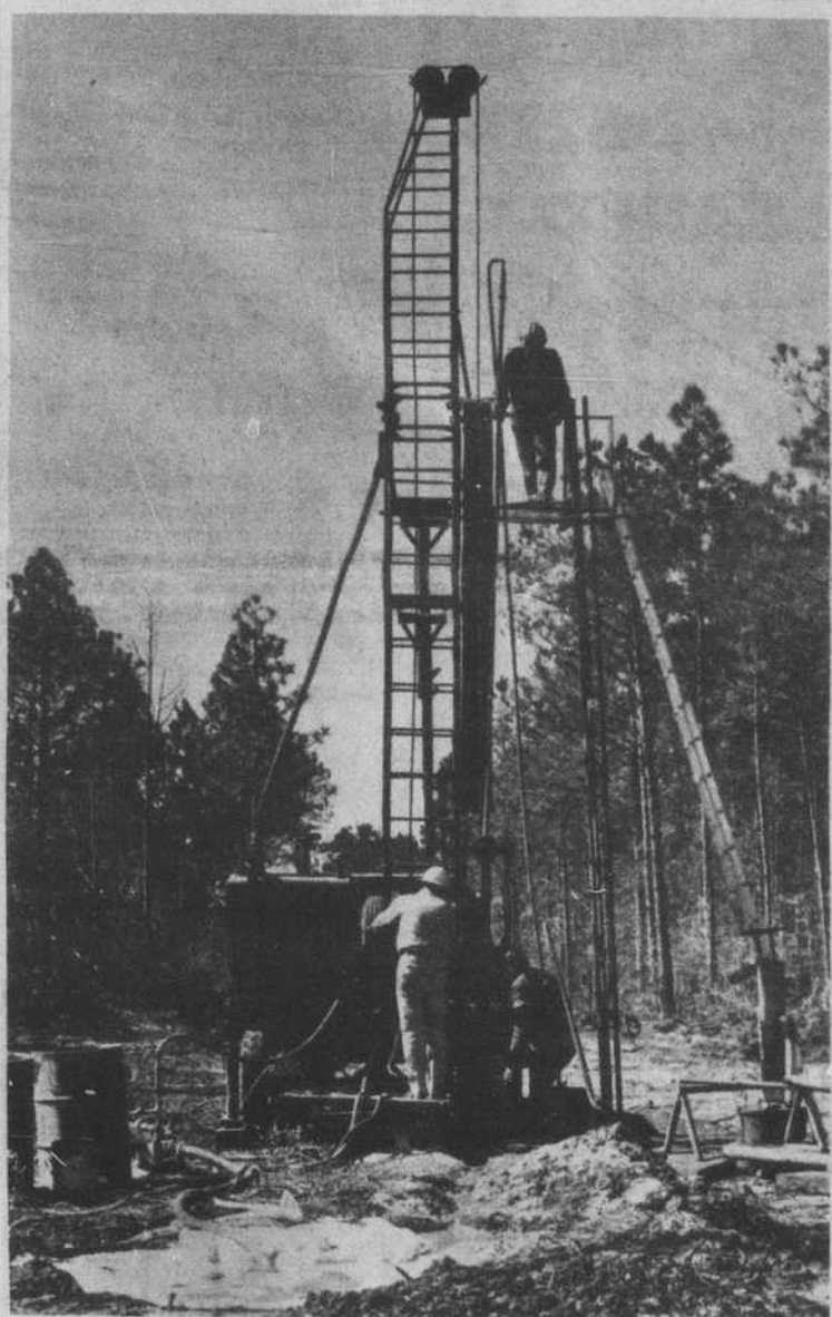
Make Test Borings
