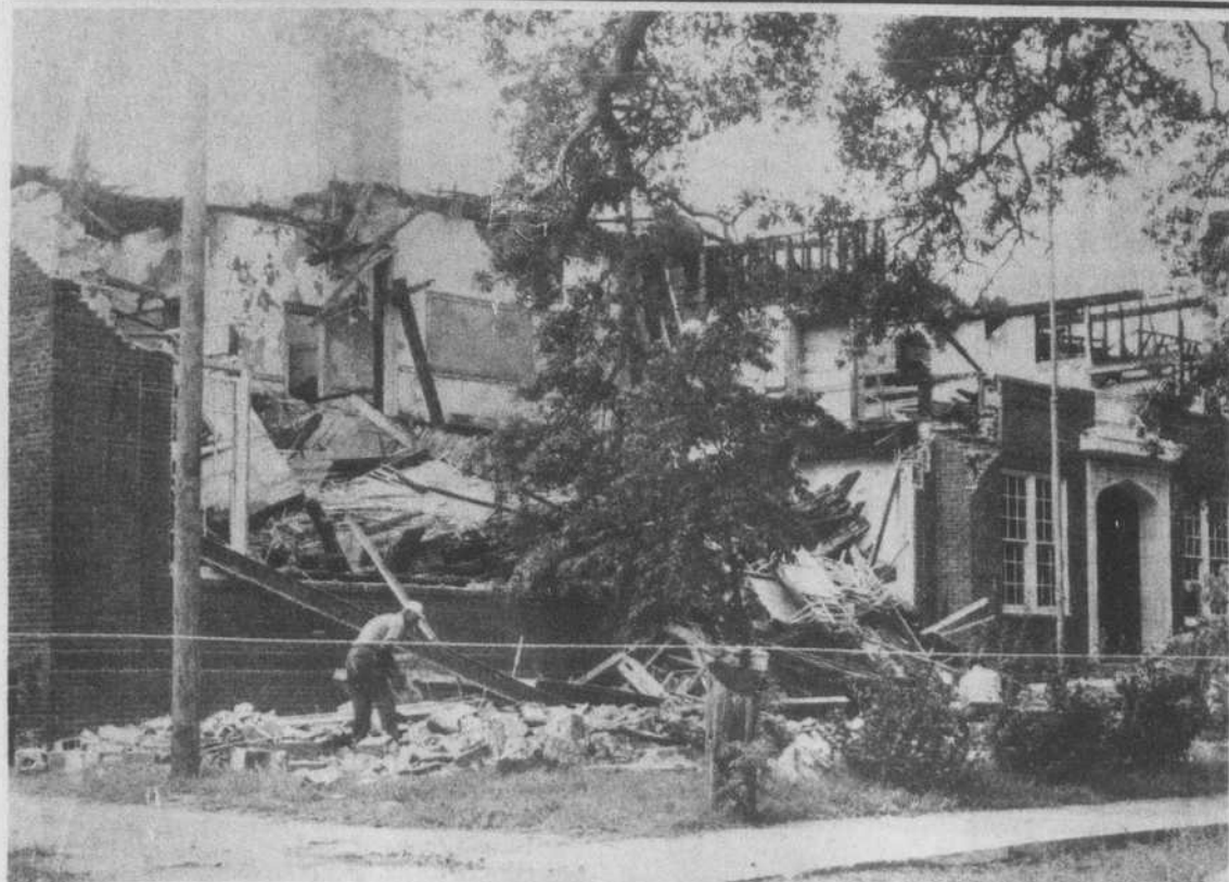
Tearing Down School
