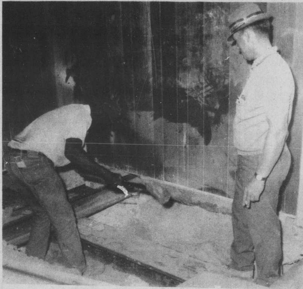
Getting Ready To Move
