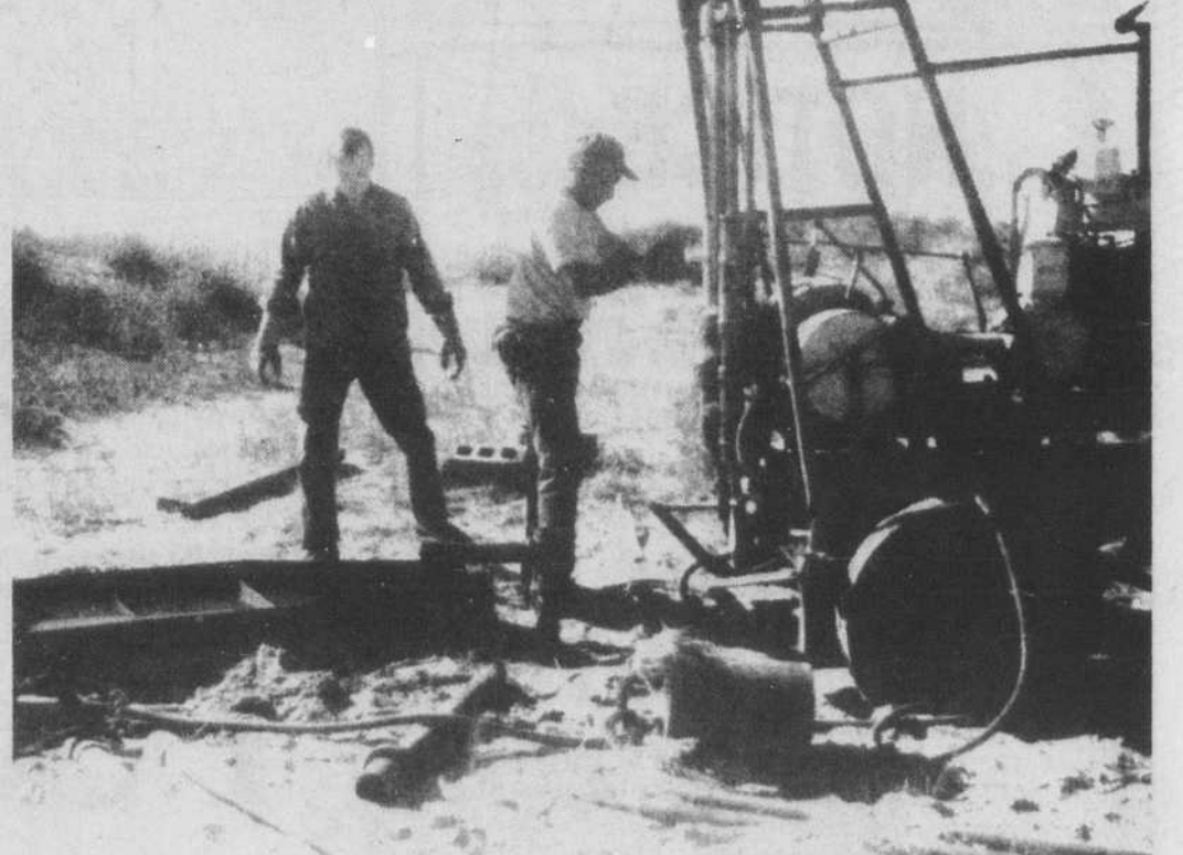
Testing For Foundation
