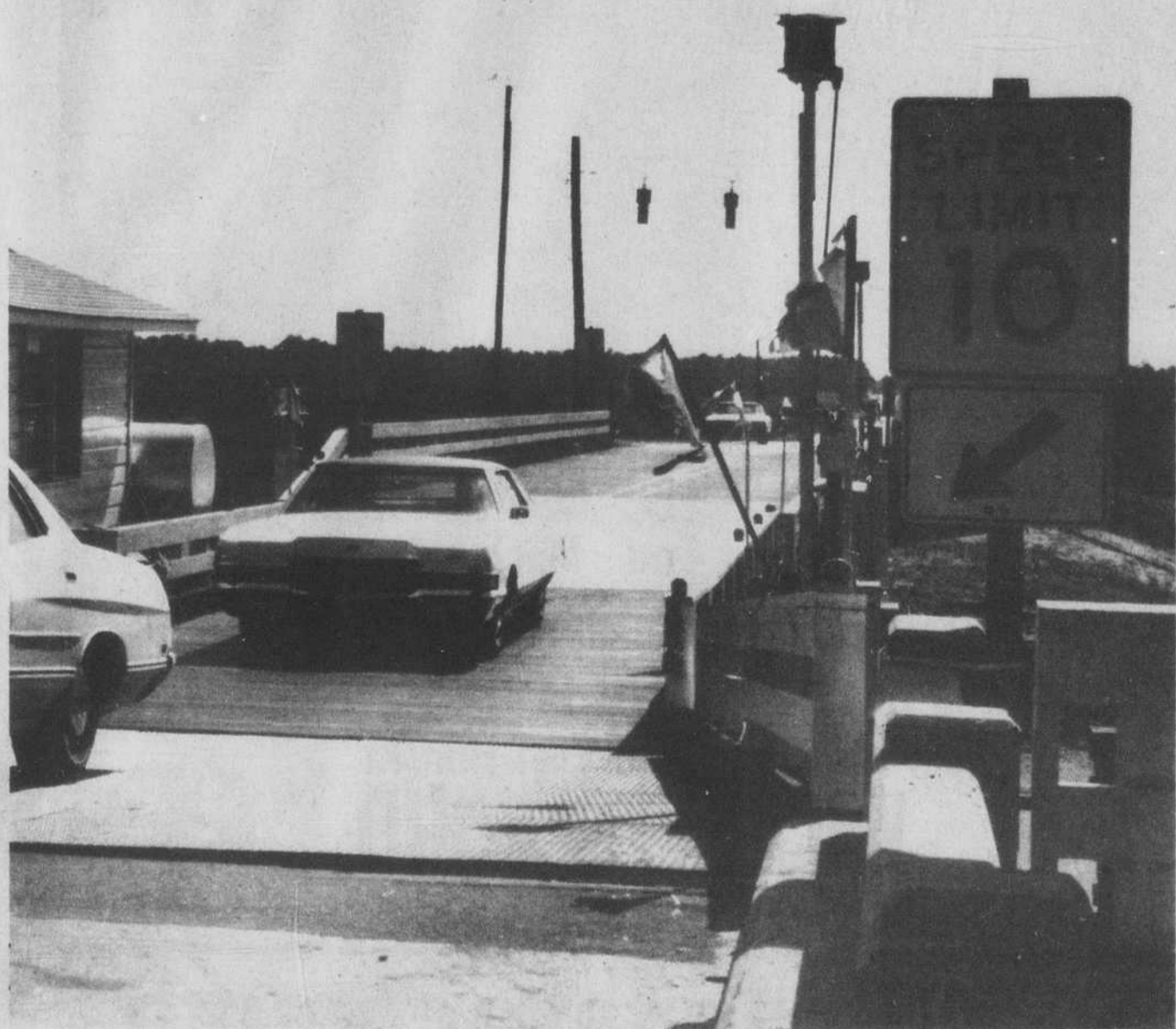
A BOTTLENECK is expected to develop this summer at this one-lane bridge, the only link between Oak Island and the mainland. The old swing-type bridge was demolished last fall by an
