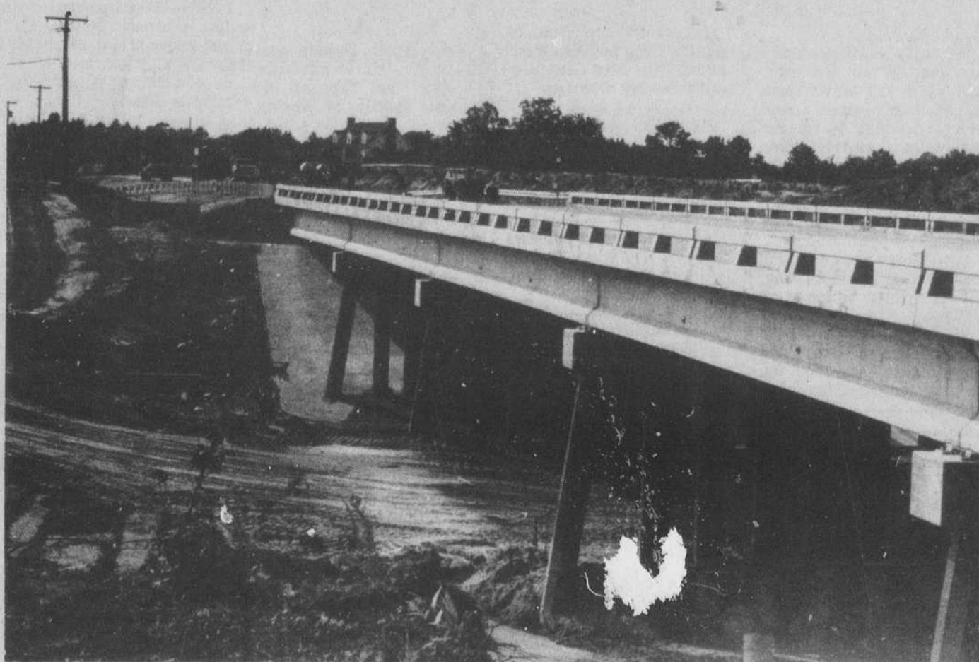
THE NC 211 BRIDGE across the Carolina Power and Light Company canal near Southport should open Thursday morning, providing a second route to town and eliminating much of the
