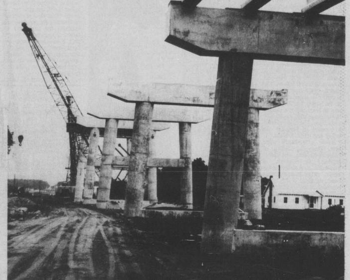
CHANCES SEEM BETTER every day that the high-level bridge to Oak Island will be completed by June 1, 1974 — the opening date set by the State Highway Commission. On the north side of the Intracoastal Waterway this construction is un-derway, while on the Oak Island side work is progressing well on the elevated causeway that will serve as the southern approach. The highlevel span will be fixed and will not open for waterway traffic, providing an uninterrupted flow of traffic on and off the Island.
