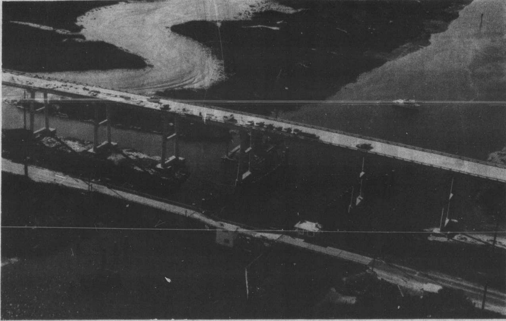
ALMOST... the "missing link" between the Southport area and Oak Island is nearing completion, evidenced by this aerial of the old (one-lane pontoon bridge) and the new (high-level structure). Note the protection for the center two supports of the new bridge.
