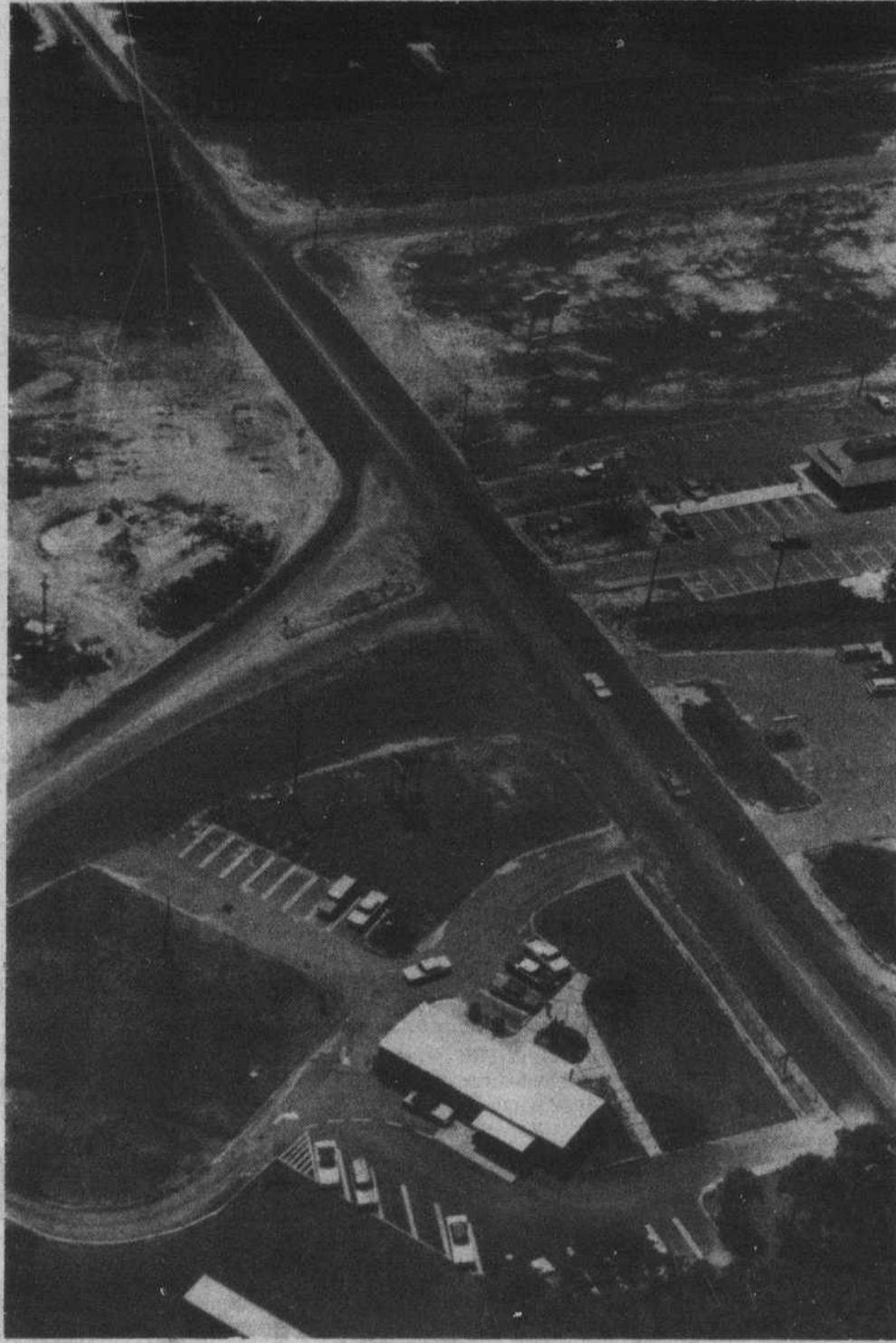
IMPROVEMENTS ARE being made to the Sawdust Trail intersection of NC routes 211 (extending from upper left to lower right of the photo) and 87. Work involves the widening of both routes to include turning lanes and, according to officials in the Department of Transportation, traffic signals.
