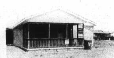
712 W. BEACH DRIVE. 3-bedroom, 2-bath second row home in great location and affordable! Remodeled, stucco exterior, and screened porch. $74,500.
