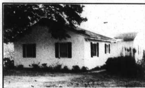
120 RIVER ROAD. A million dollar view from a fabulous fifties beauty! In need of restoration, but on the highest and largest lot on the Cape Fear River. $290,000.
