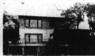
AWESOME! Impressive place for parties and weekend guests. Two-story, 4-bedroom brick house with private decks, screened porch, large rooms with solid wood trim, private boat dock on Davis Canal on two beautiful wooded lots. Garage with separate storage room. This gorgeous home is only $198,000.
