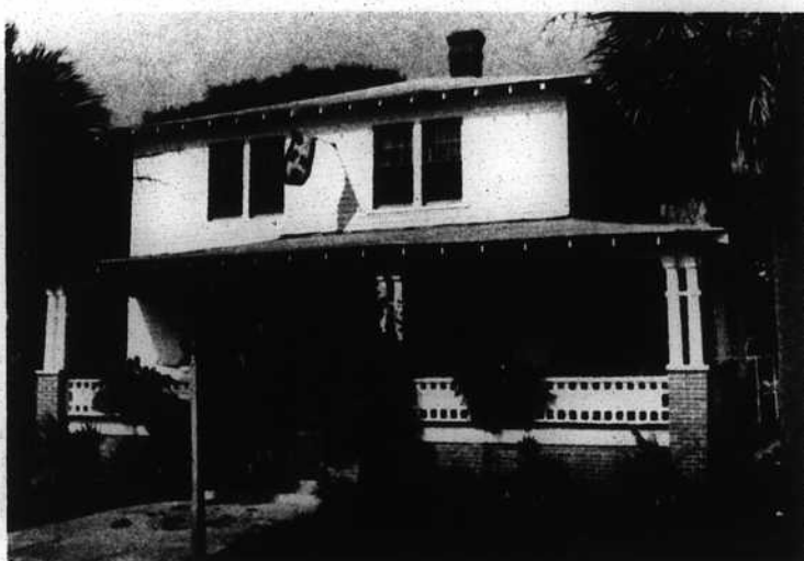
202 WEST BAY STREET
