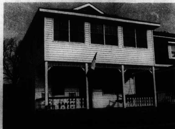
114 WEST BAY STREET
