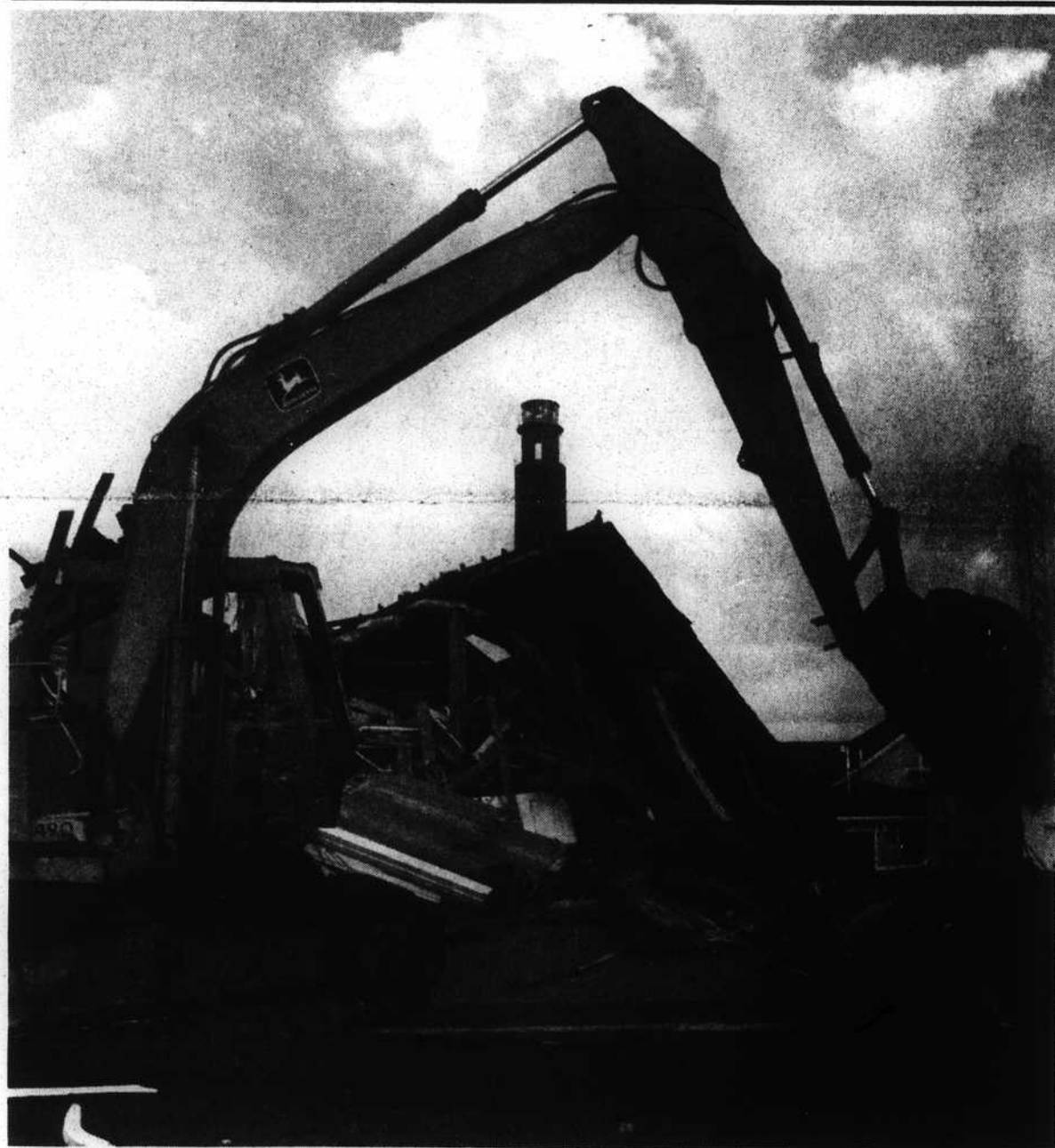
In a matter of minutes last week a wrecking crew reduced the former headquarters of Oak Island Coast Guard station -- a large, white, imposing structure -- to rubble. The old building was supplanted last year by a modern one, seen in the right background.
