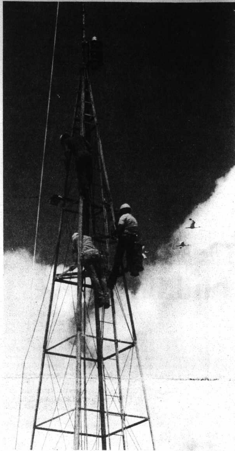
Photo by Jim Harper City workers got a bird's-eye view of the waterfront last week as they prepared to replace the damaged wind-vane atop the weather tower on the Garrison. The device that weathered the March 13 storm suffered in a later entanglement with a flag.
