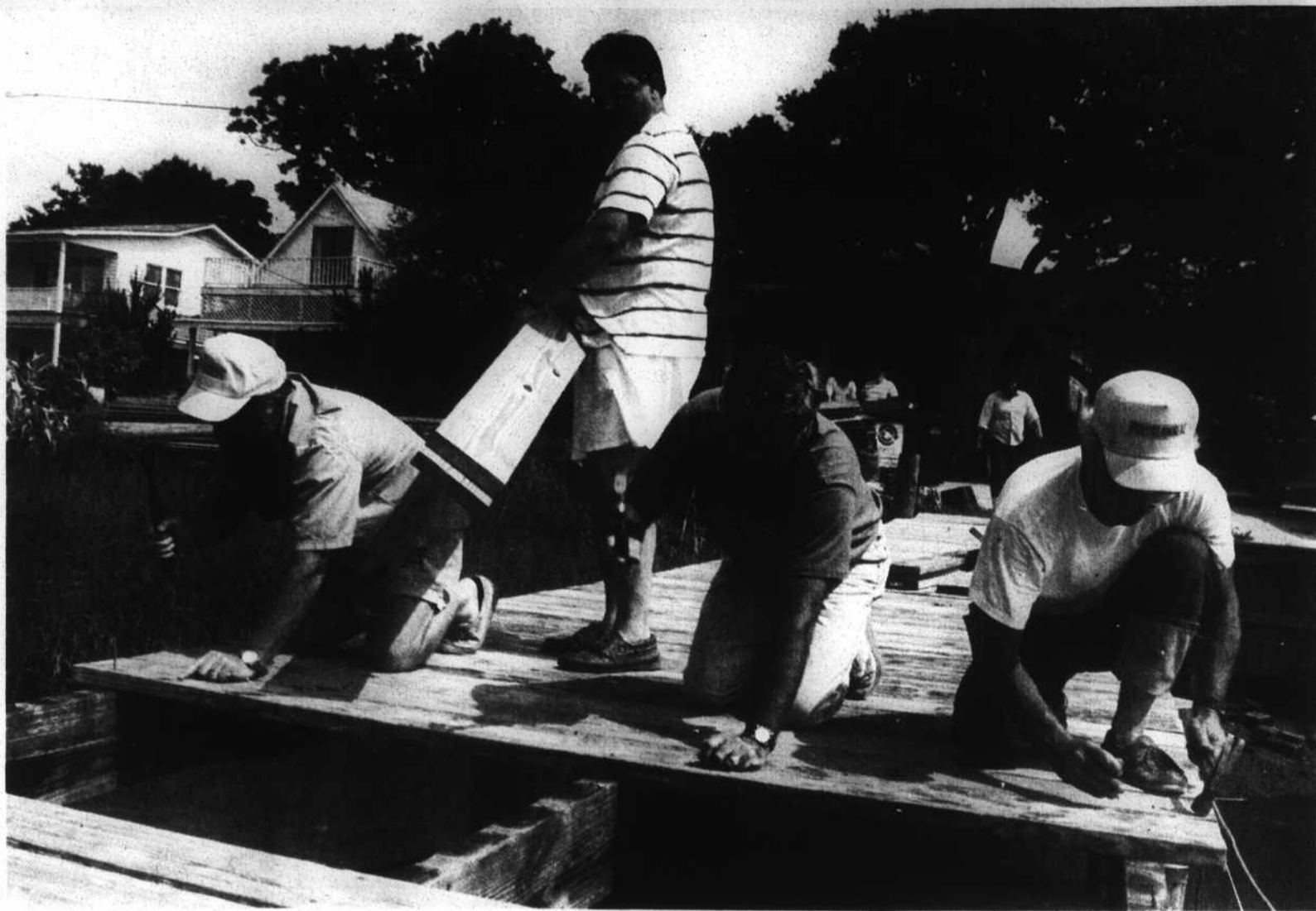
Southporters hammered in the morning on Saturday, repairing the city dock at the west end of the yacht basin. Mayor Norman Holden (center) helps install one of the planks donated by private citizens. Other planks were provided by makers of the movie "Birds II".
