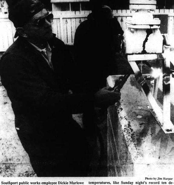
removes a cracked valve from the city's water tank Monday morning after sub-freezing temperatures ruptured the uninsulated valve. The city installed a new, insulated valve that will withstand low
