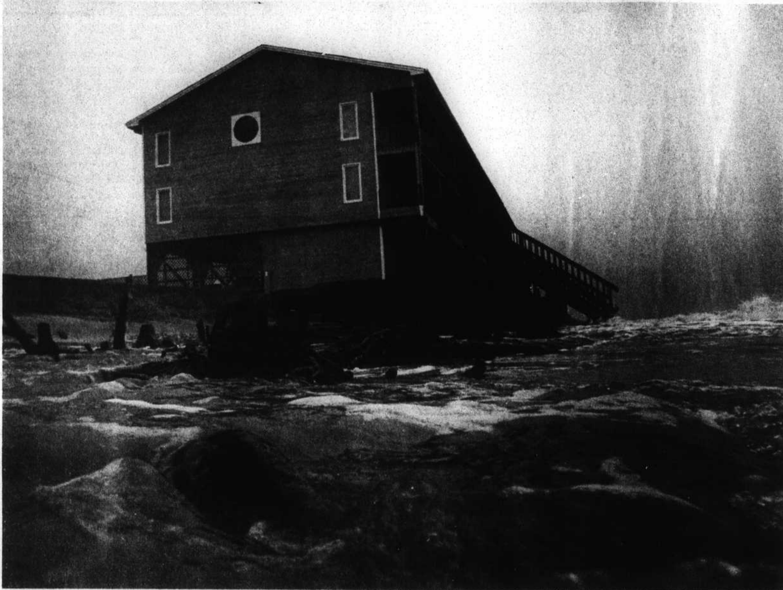
Sea Horse townhomes at 4611 East Beach Drive in Long Beach, already threatened by winter erosion, were severely undercut by wind-driven high tides last week that exposed long-buried tree stumps and
