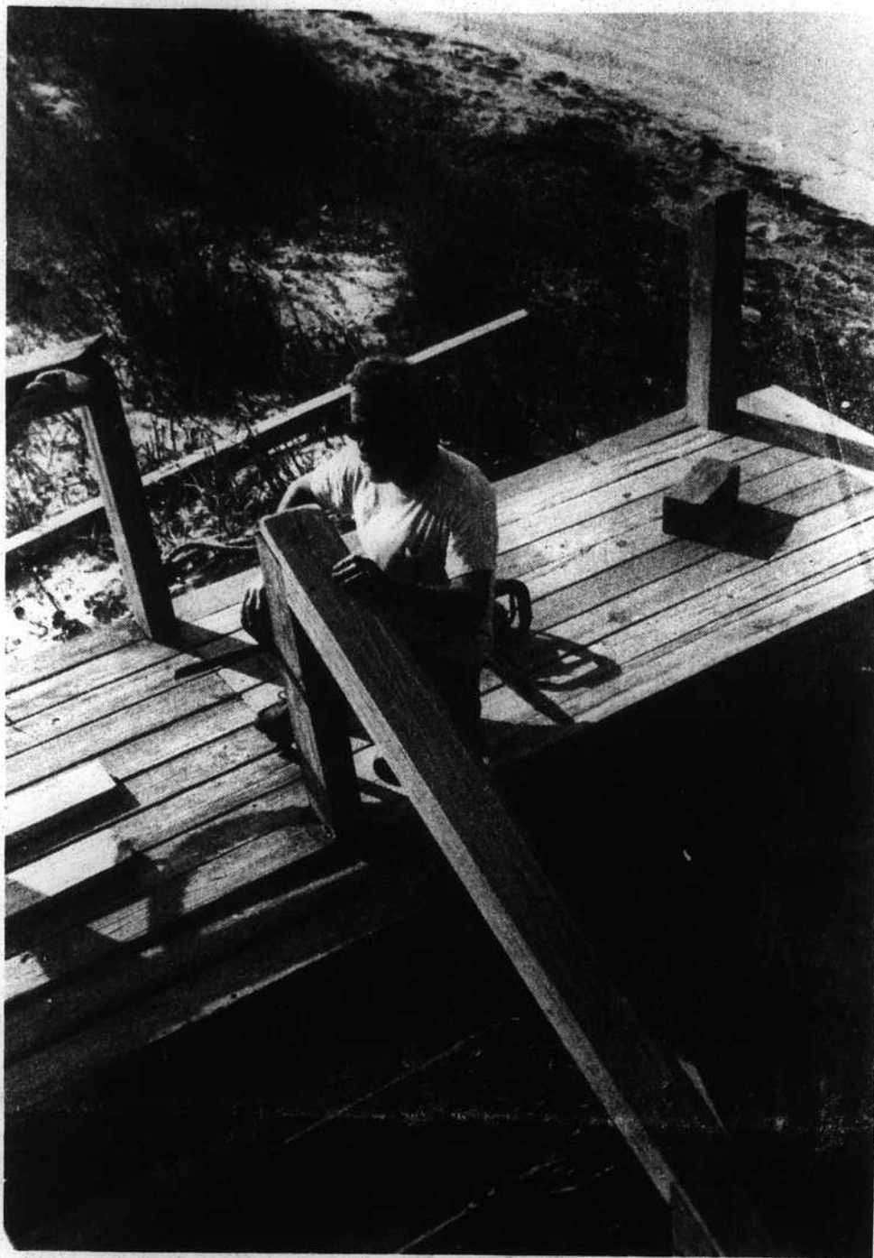
While erosion is a common concern on Oak Island, significant accretion has occurred over the past several years at each end of the island. Sand has buried many waterside steps near the east end of Caswell Beach, and on Monday Phil Tate was extending his deck there and adding new steps to the strand with the approval of coastal management authorities.
