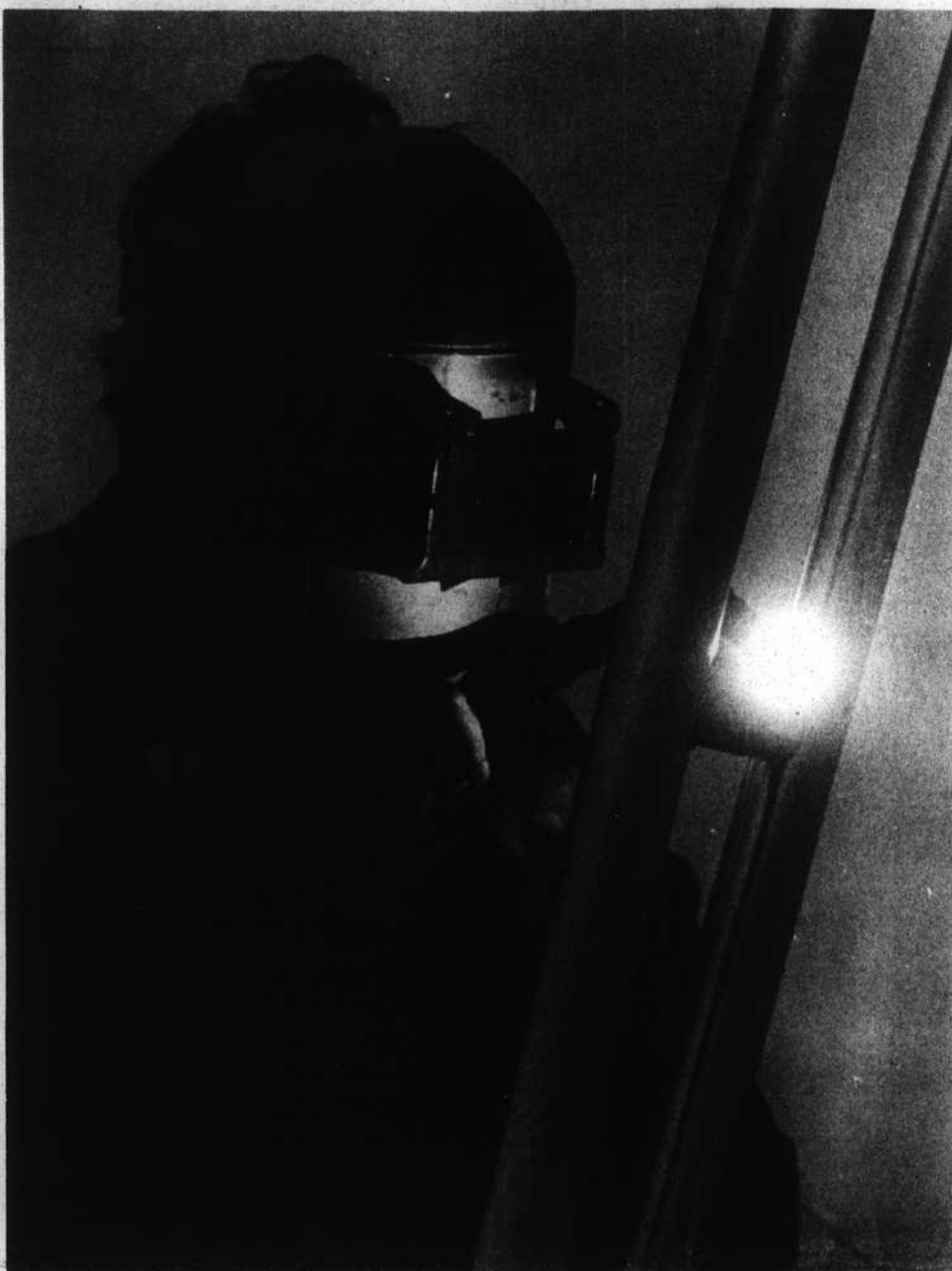
Photo by Jim Harper Pipewelder Tim Ehling found both light and shelter on a murky, misty morning recently to get his work accomplished. He was welding on the bridge of a new sports yacht in the Southport yacht basin.
