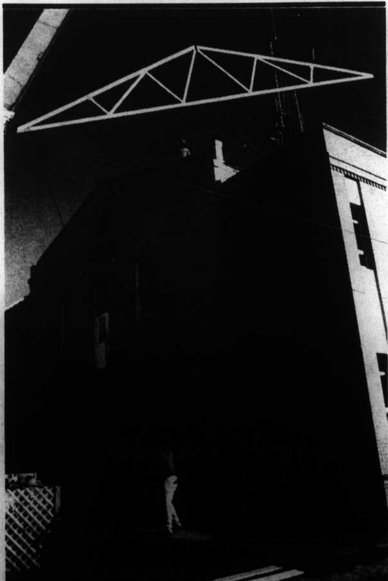
Work continued this week on repair of the leaky City Hall roof. It is hoped by installing a pitched roof on the building a repeat of the damage caused by Friday's storm will be avoided. Water poured inside City Hall, flooding the old courtroom upstairs and damaging records and carpeting on the ground floor.
