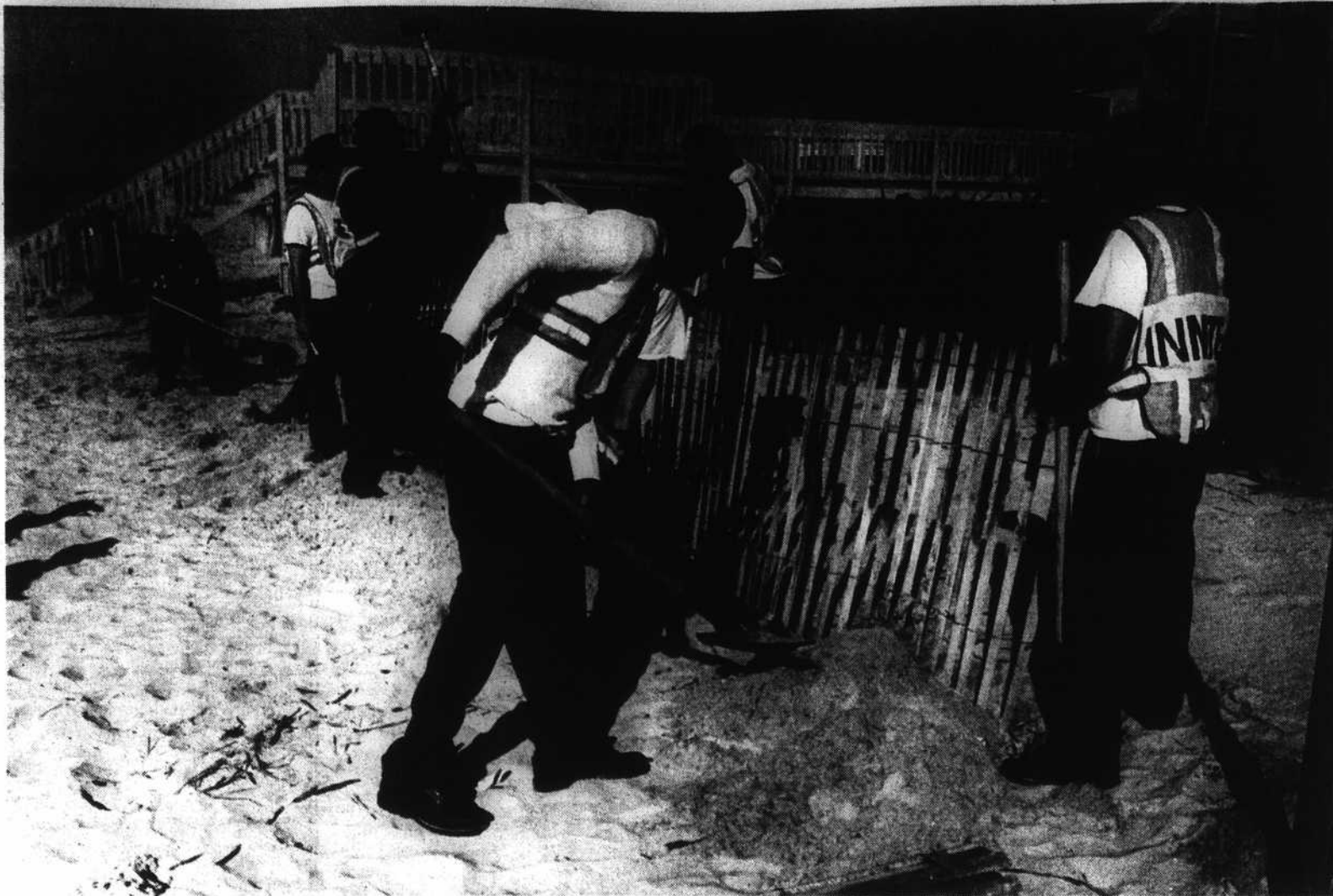
Inmates from the N. C. Department of Corrections unit at New Hanover County Monday installed experimental dune replenishment fencing along a 1,200-foot stretch of Caswell Beach, beginning at the
