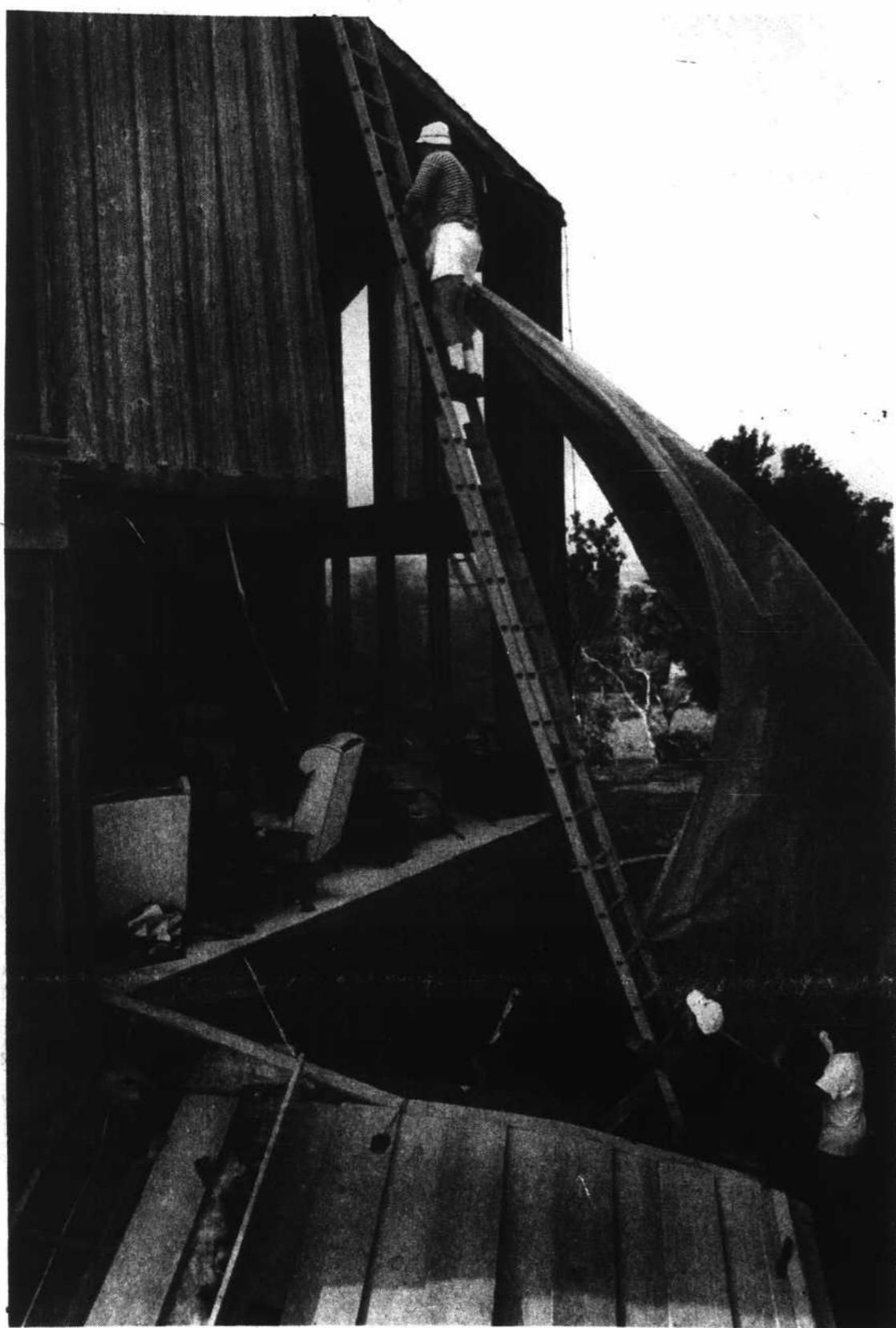
Photo by Jim Harper Bill Boyd -- "doing what neighbors do" -- rigs a tarpaulin to cover the bared side of Ralph Whitesides' Caswell Beach living room Saturday with the help of police chief Paul Osborne and Randy Whitesides. This damage was extraordinary in a storm which generally caused little property damage and no reported major injury in the community.
