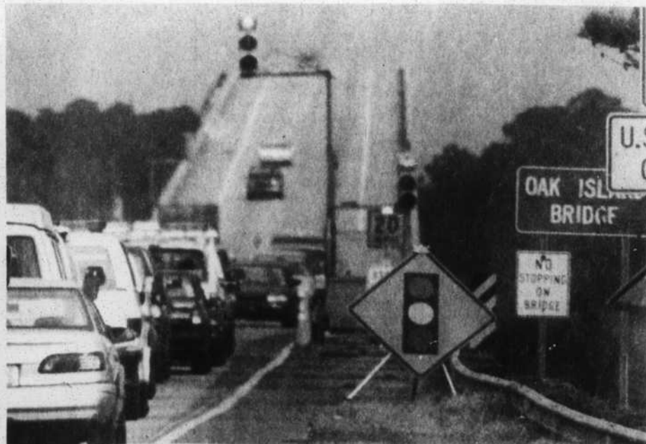
Traffic backups on the Oak Island bridge were annoying at times this week as the N. C. Department of Transportation began routine replacement of bridge joints. In place of flagmen, DOT employed portable traffic lights to narrow traffic to one lane across sections of the bridge as work progressed.
