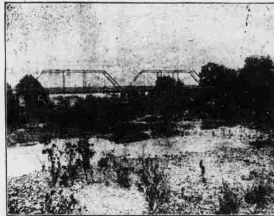
Bridge Across Deep River at Island Ford
