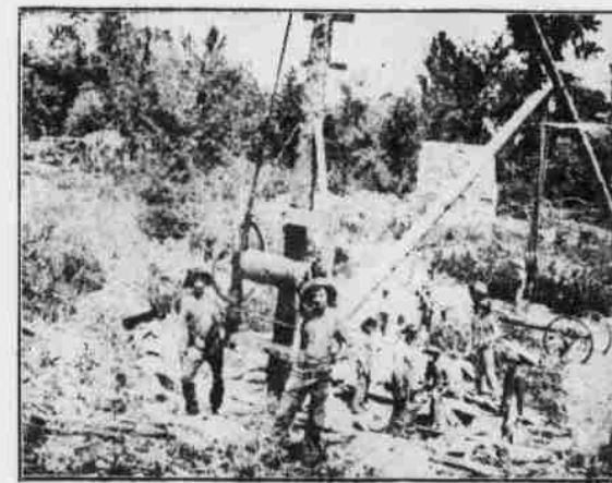
Building Bridge Across Richland at Moffitt's Mill
