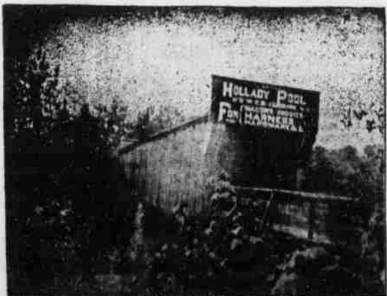
Bridge Across Bruah Breek at Cheek's Mill
