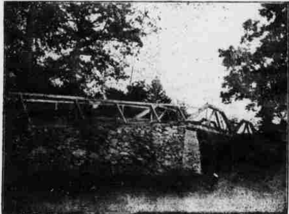
Bridge Across Little River at Williams Place
