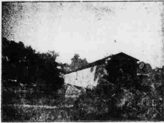
Bridge Across Deep River at Randleman
