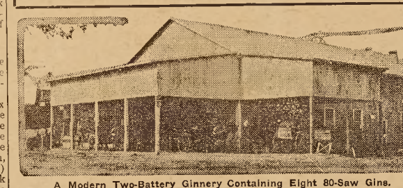
A Modern Two-Battery Ginney Containing Eight 80-Saw Gins.
