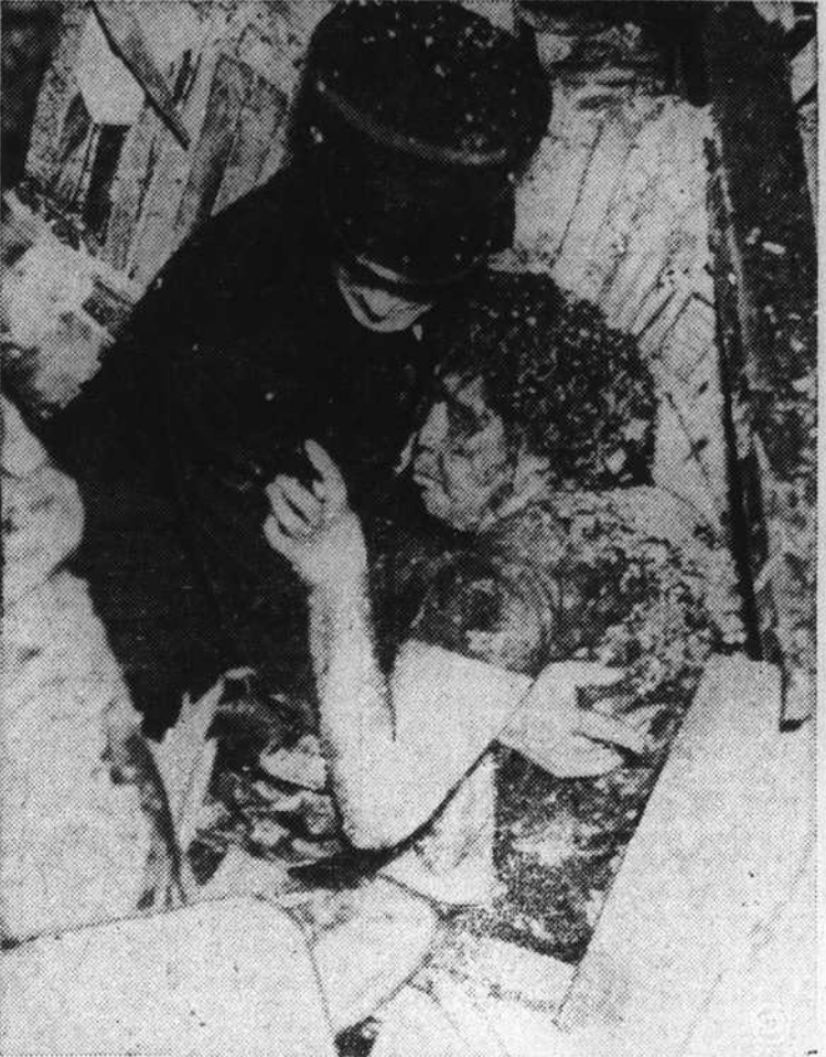
Mutely, pathetically Marie Coral clutches at the arm of the fireman who strives to drag her from the wreck of the New Brighton, S. I. tenement house in which she was trapped by collapse of the building. Her hair and back are covered with fragments of plaster and she has several internal injuries in the disaster which killed 11.
