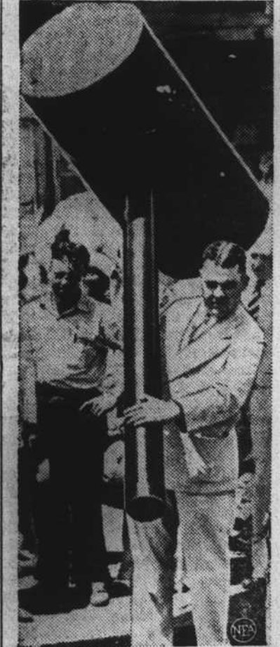
Taking a huge sledge-hammer in hand, Gov. Richard W. Leche of Louisiana is shown above as he prepared to drive the first piling for the new $10,000,000 toll-free bridge to be built across the Mississippi river at Baton Rouge. Scheduled to be completed in 1939, the bridge proper will be 2 1/2 miles long, with the approaches making it a five-mile project in all.
