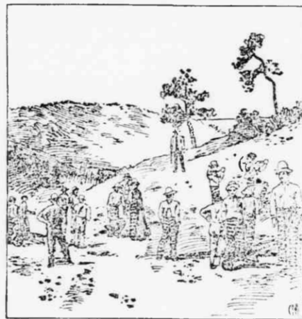
CONVICTS AS ROAD WORKERS.
