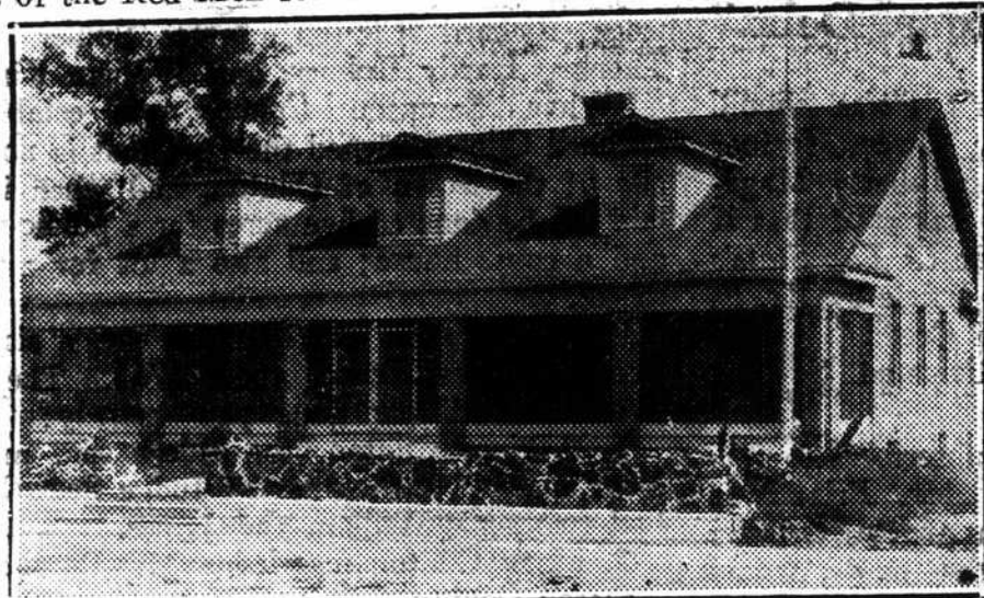
THE CLINTON COMMUNITY BUILDING.
