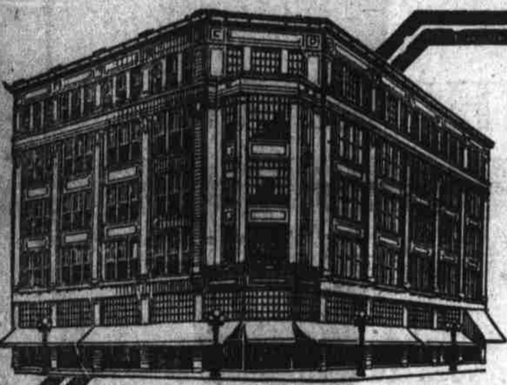
Saks Building, Birmingham. Carey Roofing Used.
