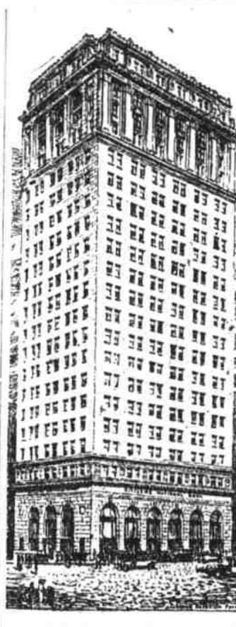
The Citizens National Bank of Baltimore now under construction.
