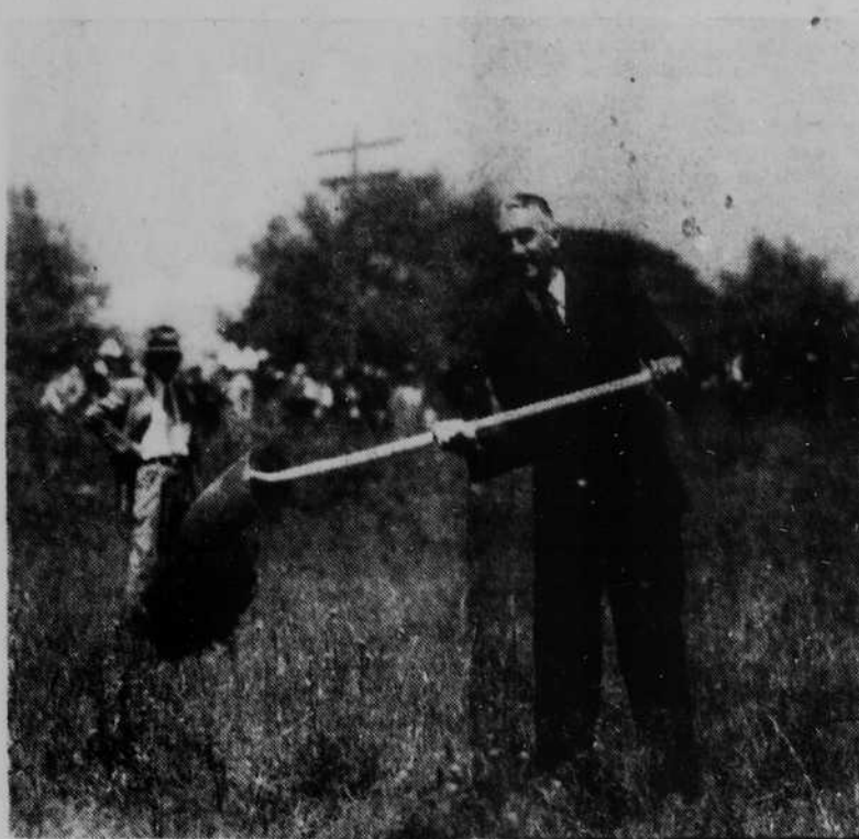
Shown here is Ralph H. Ramsey, Jr., chairman of the board of trustees of the Transylvania community hospital, as he turned the first shovel of dirt for the new $86,000 hospital building. Actual construction work is getting under way this week on the new building.
