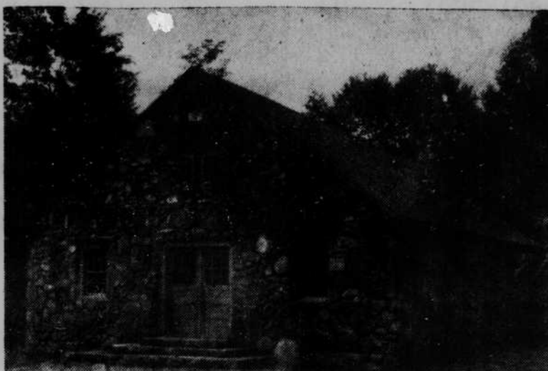
Above is a view of the new English Chapel which has just been erected near the Davidson River just off the Trans-Pisgah Forest highway about four miles from Brevard. It is constructed of native stone gathered from the Davidson River.
