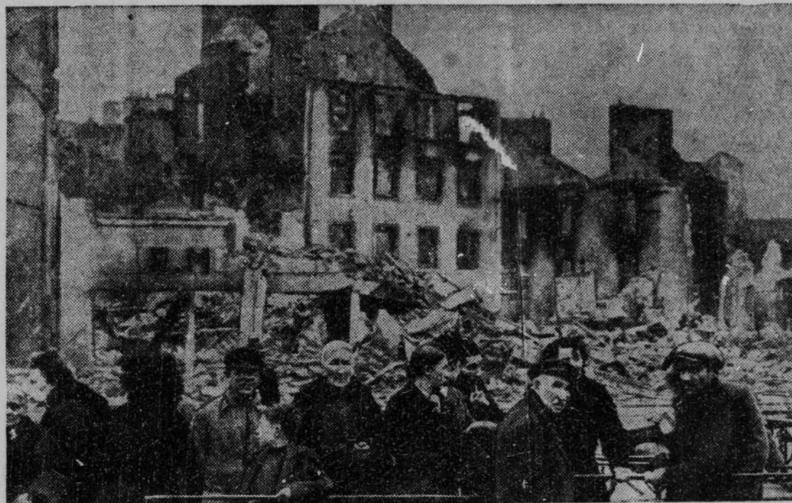
AMERICAN AND BRITISH BOMBING ATTACKS on the Nazi sub base at Lorient, France, have left their mark on the city. This photo, published in a German-controlled magazine, shows some of the buildings wrecked by the Allied blitzing. Damage to the submarine pens is not mentioned by the Nazis. According to the French caption, the people in the foreground are said to be evacuees. (International)
